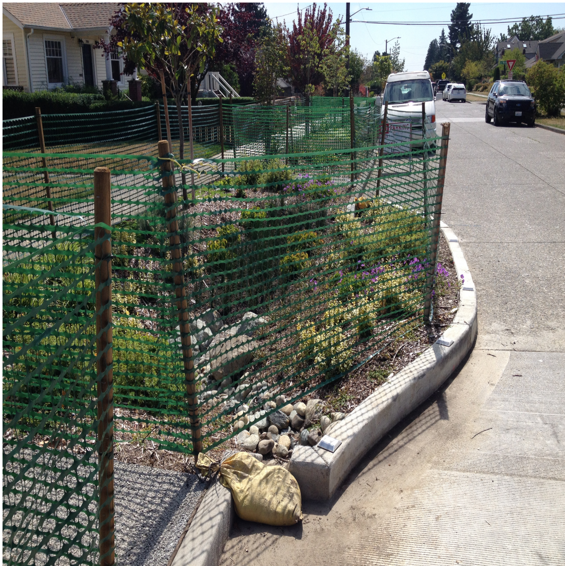
Sand bags prevent silt-laden flow from entering the bioretention BMP. Green construction fencing prevents compaction due to foot traffic.
