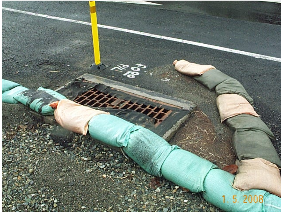
Temporary sand bags divert construction site stormwater runoff to inlet protected with a catch basin filter sock.
