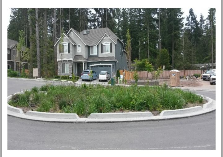
Bioretention BMP in a cul-de-sac of a LID residential neighborhood in construction in western WA. The bioretention manages stormwater runoff from the roadway and contributing roof and driveway areas. Numerous large existing trees were retained, adding valuable stormwater and community benefits.
