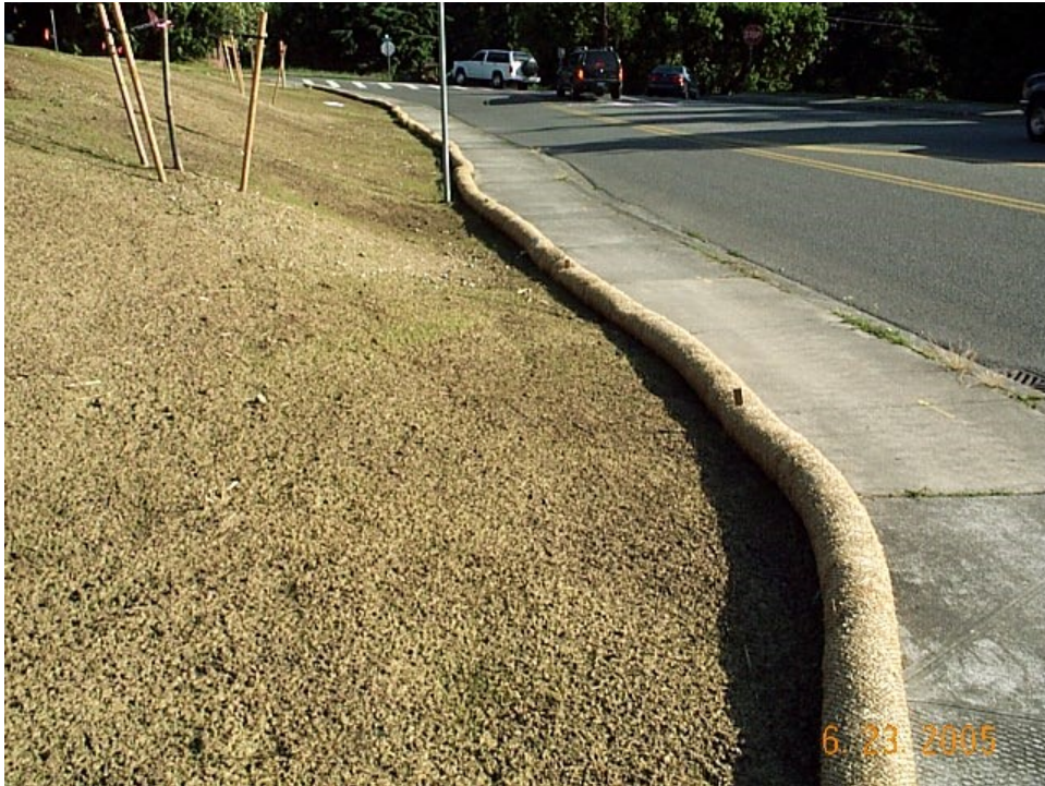
Example of shallow gradient slope with berm installed at downgradient edge to minimize silt-laden runoff onto the sidewalk.
